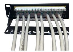
6. Secure the cables to the cable management bar using cable ties, taking care not to over tighten them.
