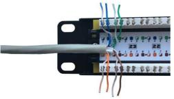
Punch down the wires using a Krone type or 110 style termination tool.
